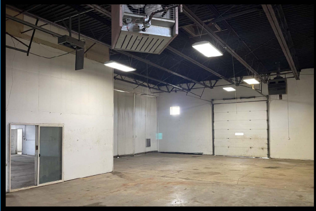
South Overhead Door
