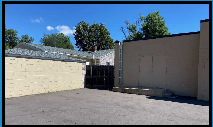
Exterior Loading Doors
